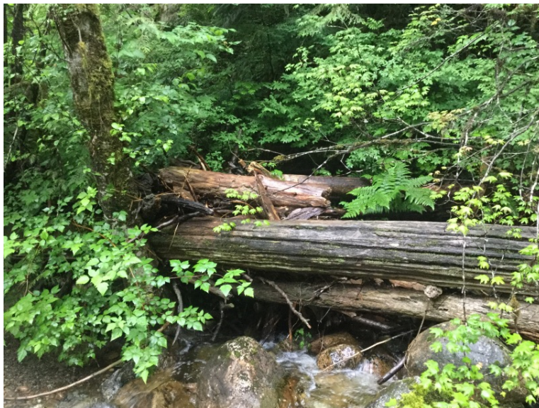
Debris accumulations at inlet
